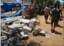
The front wall of the hospital destroyed in the attack
